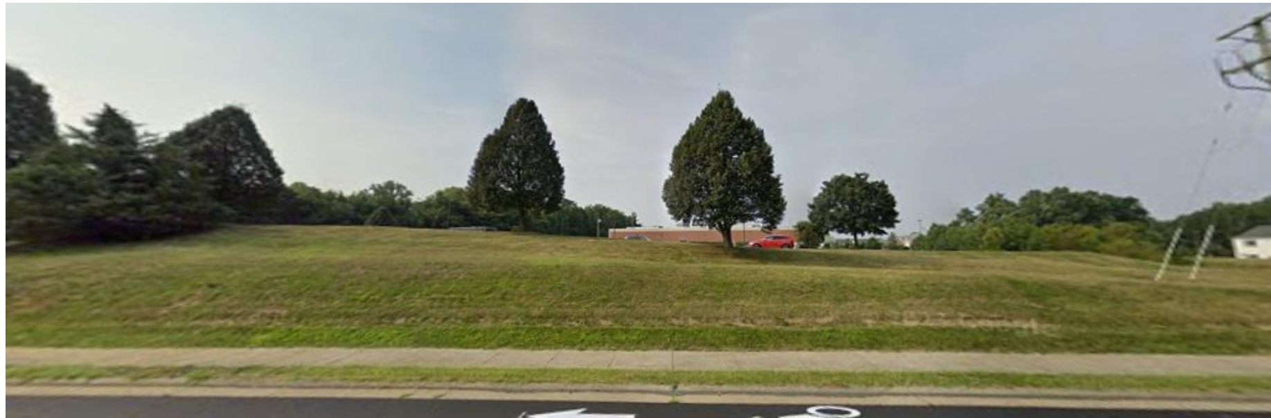
Figures 3a-b: Views of the existing building from the Airport Road Entrane Corridor.
